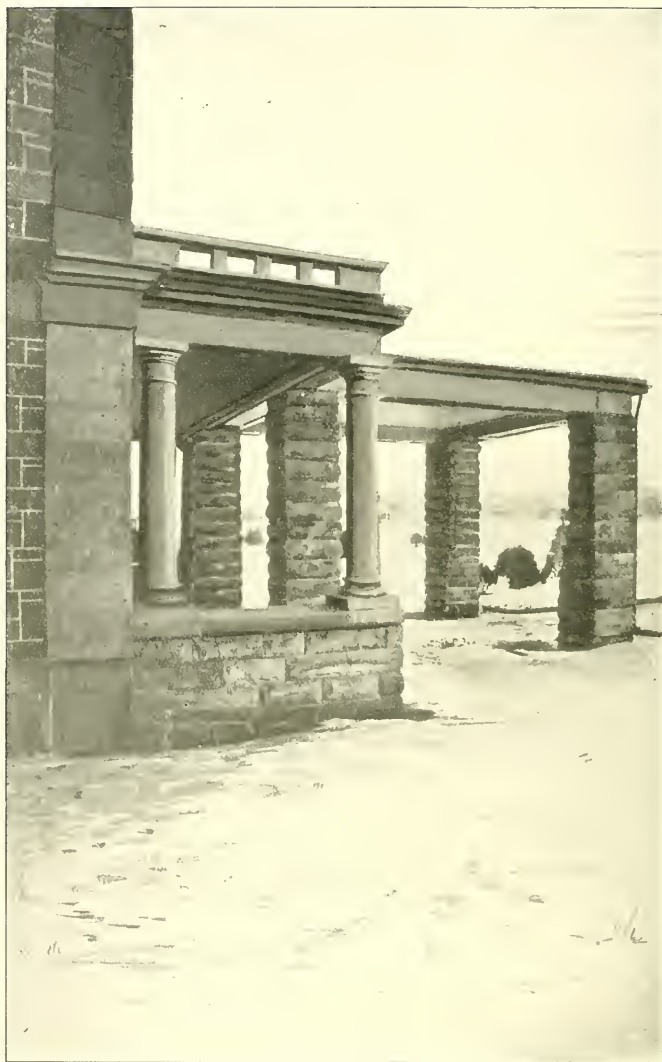
Front Entrance to the Hospital, Warren.
